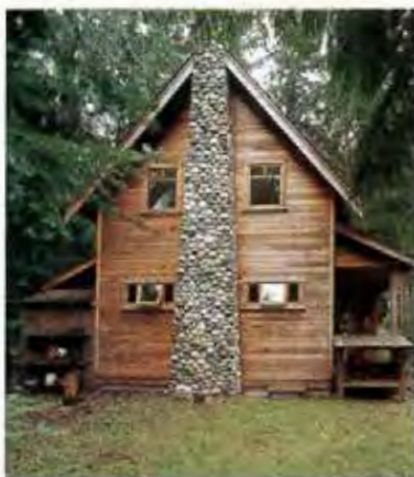
▲ Like the slender, tapered trunk of a Douglas fir tree, this mosaic rubblestone chimney reaches to the sky. Combined with the horizontal siding, the thin taper accentuates the steep peak of the gable.
