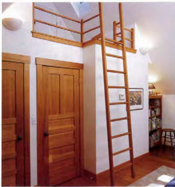
△ The woodwork in the children's bedroom combines usefulness, beauty, and delight. The ladder, with its wood pegs, smooth finish, and rounded ends, is a work of art that carries the kids up to the loft.
