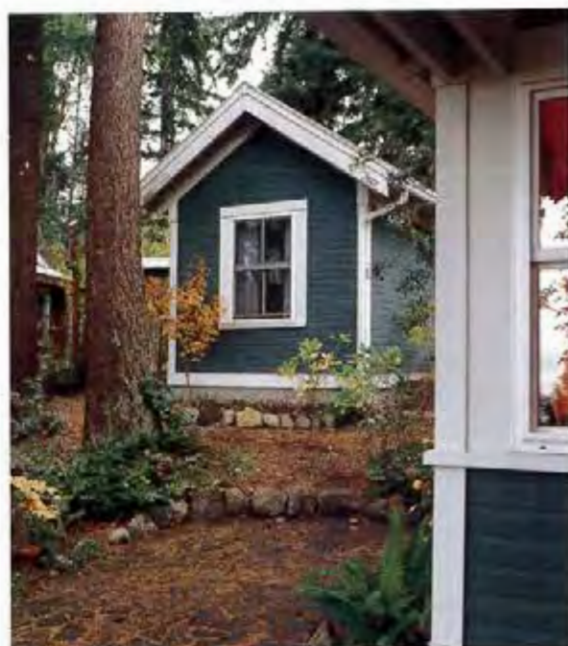
Overnight guests enjoy the intimate scale and privacy of the adjacent studio/guest cottage. Wide window trim, corner boards, fascia, frieze, and belly-band, all painted white, give the small structure the appearance of a dollhouse.
